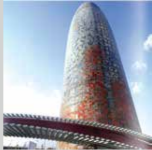
Torre Agbar, Barcelona, Spain
